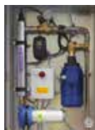
OS-ONDA SPRAY SYSTEM Air saturation 80% Air temp. Reduction 8K
