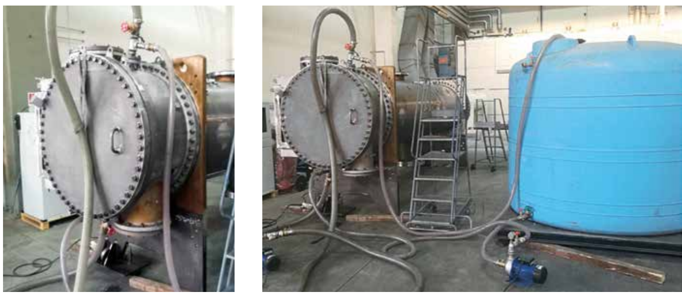
ONDA can provide the tubes passivation to prevent corrosion during the heat exchanger commissioning
